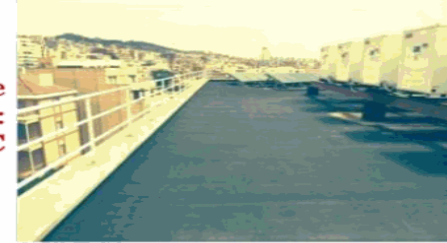
Before: Barcelona, black modified bituminous roof. 2014.
